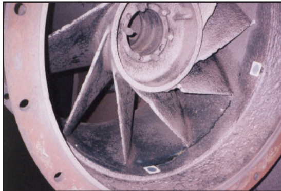
Pump condition after removal of the old coal tar coating
